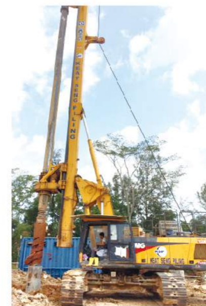
XR220D新加坡施工 XR220D working in Singapore
