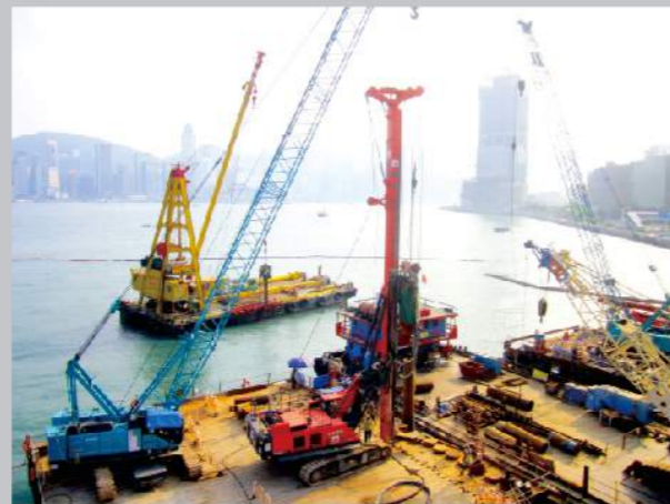
徐工气动潜孔锤旋挖钻机征战香港维多利亚港 XCMG rotary drilling rigs with DTH are working in Victoria, Hong Kong
