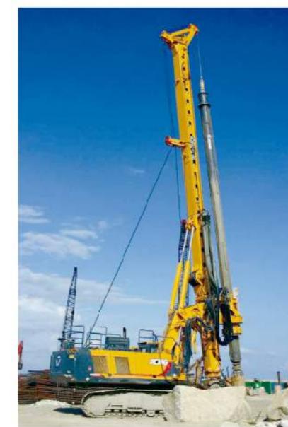
XR280DII马来西亚TERENGGANU施工 XR280DII working in TERENGGANU Malaysia
