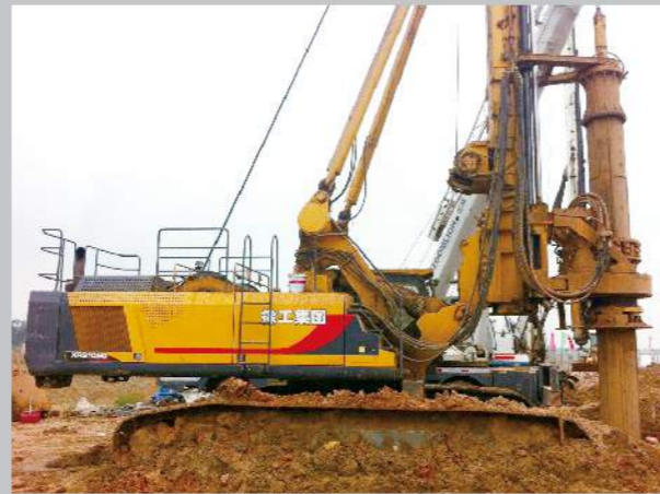
新郑机场跨航空港区南水北调工程大桥 XCMG rotary drilling rigs are working in South water to North Project
