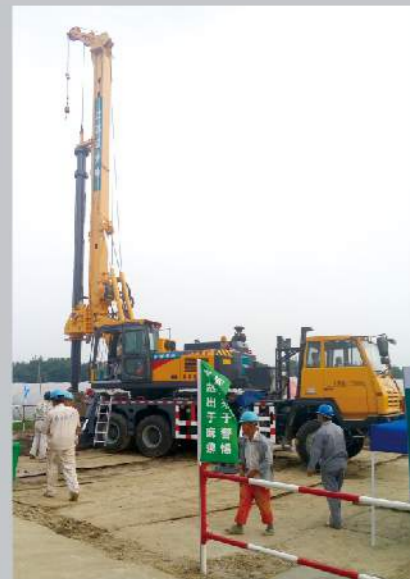
XRL100江苏送变电施工 XRL100 in Jiangsu electricity project
