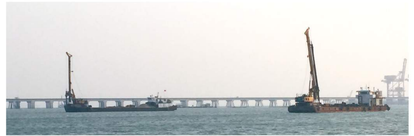
徐工旋挖钻海上展雄风 首次实现多台钻机海底成槽作业 XCMG rotary drilling rigs are making trench on the seabed
