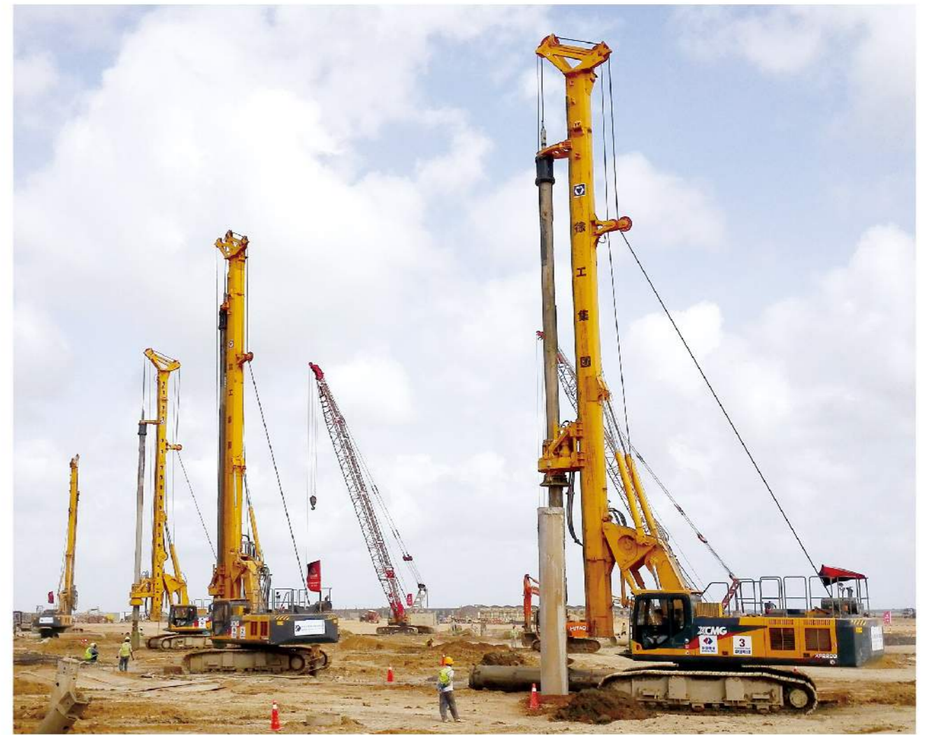
徐工旋挖钻“一带一路”显风采，群机助力巴基斯坦新建设 XCMG rotary drilling rigs are working in One Belt, One Road project in Pakistan
